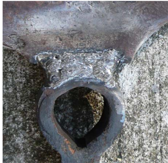
Figure 4: Anvil welded to post.
