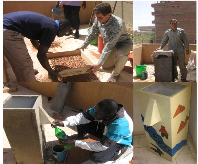
Bio Sand Filter Construction
