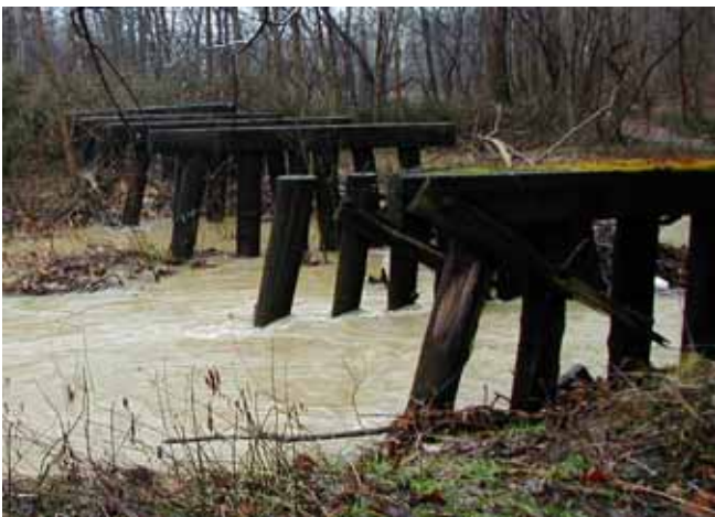
Future Stream Crossing for the Covered Bridge Gateway Trail
